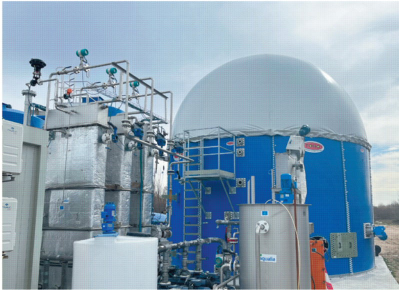
FIGURA 2. BIORREACTOR ANAERÓBICO Y SET DE MEMBRANAS FIGURE 2. ANAEROBIC BIOREACTOR AND MEMBRANE SET
